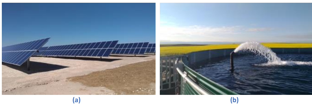
Figure 11 – Stand-alone PVIS in Alaejos, Spain: (a) 160 kWp PV generator; (b) intermediate water tank.
