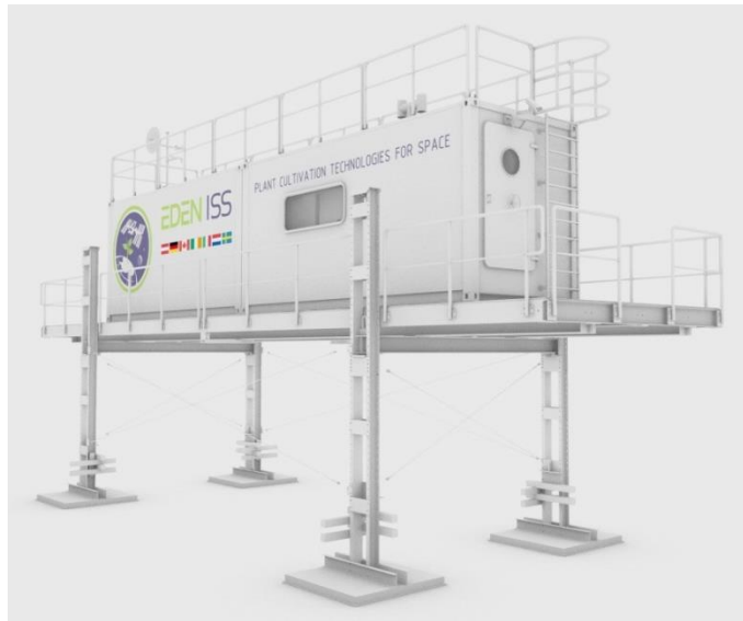
Figure 6. Illustrative impression of the EDEN ISS Mobile Test Facility mounted on the elevated platform (note that the image shows the complete platform, the bottom half of the pillars will be buried in the Antarctic ice) (Credit: Liquifer Systems Group).
