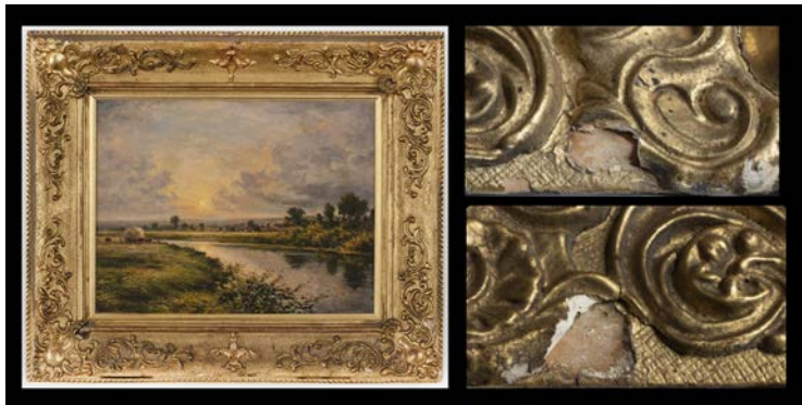
Figure 7.29: One of the recovered paintings (left), and two regions with part of the frame missing (right)
