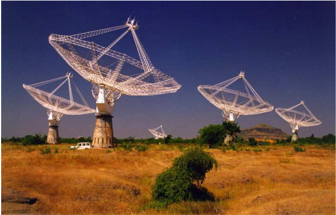
Figure 2.11: The GMRT antennas, illustrating the light-weight construction of the dishes.
