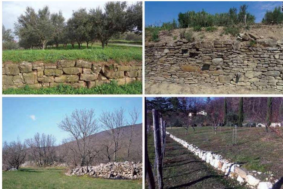
Fig.2 Terraces with olive groves and dry stone walls in Krkavče and Strunjan; terraced pastures in Podgorje in the Karst area; and old vineyard and orchard terraces in Kamnje in the Vipava Valley (all Lučka Ažman Momirski)
