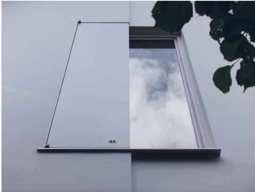
The mirror shutters of the built version of the project retained several features of this device while enriching it. In the closed position, their outer face was as naked as the wall and picked up the colour and the smooth, matte materiality. In a semi-open position, their oblique orientation contributed to the strategy of connecting and circulating the elements of the house.
