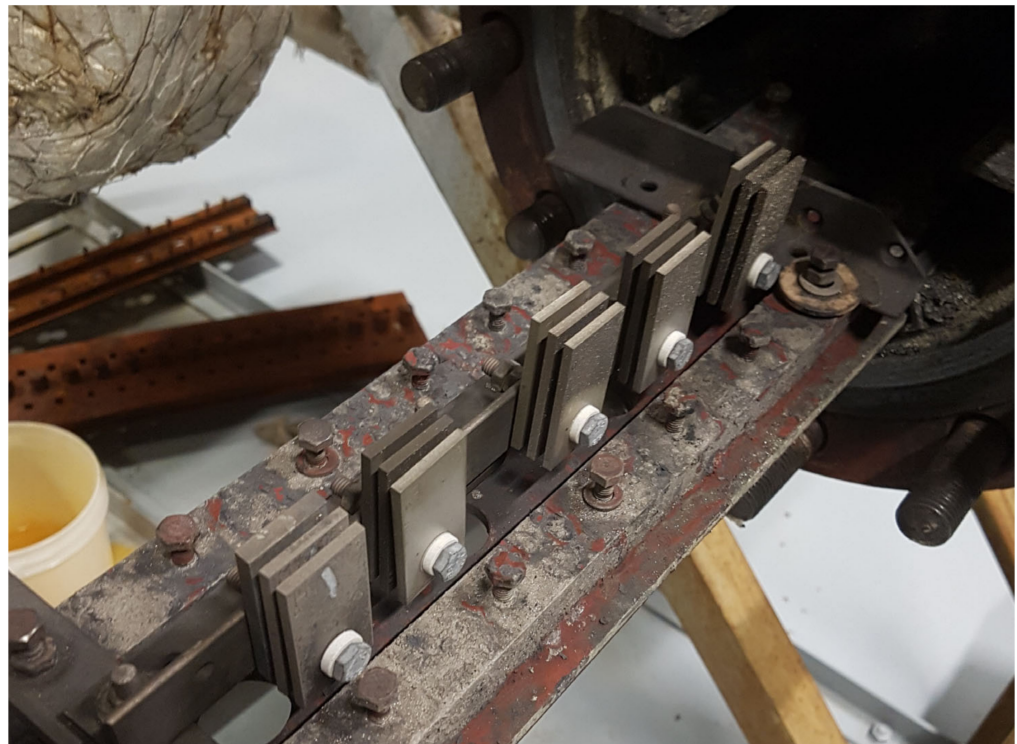
Figure 3. The coupons being removed from the pressure vessel at Reykjanes power plant where they were exposed.
