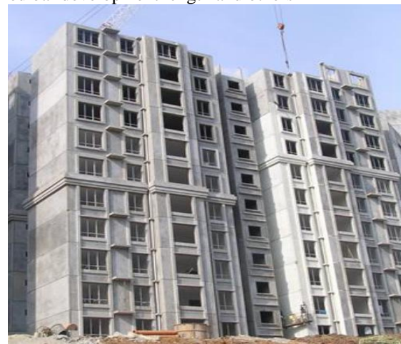
Fig. 1 : Precast Concrete Building
