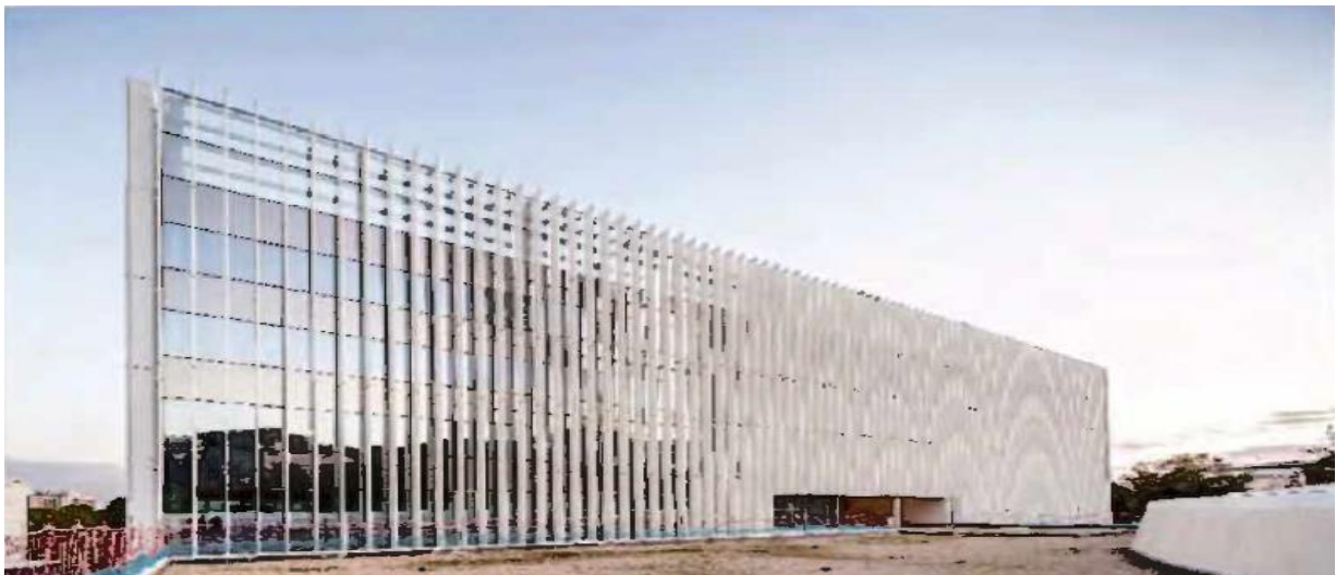
Figure 3. BSC new headquarters
