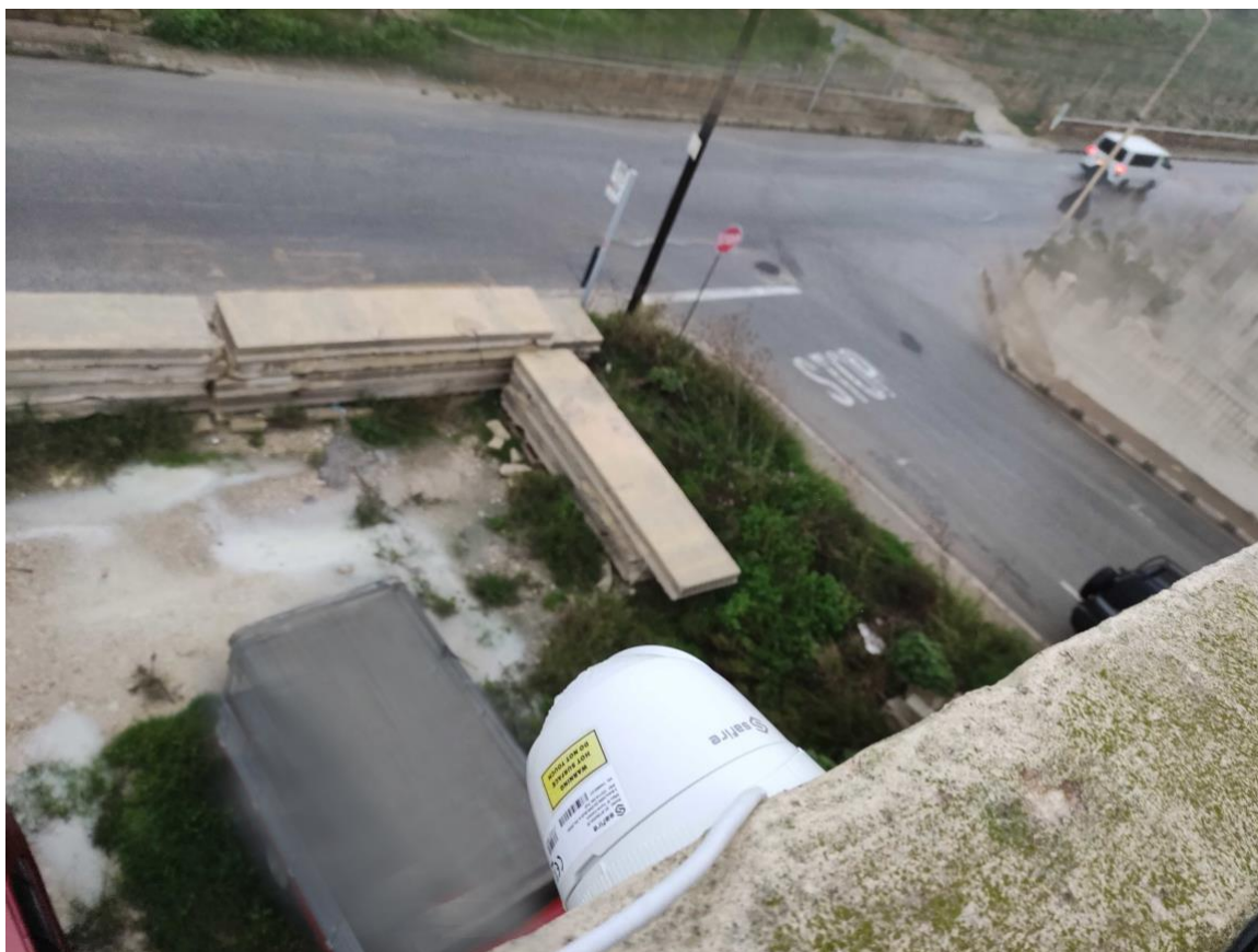
Figure 3. Image of camera used to inspect junction
