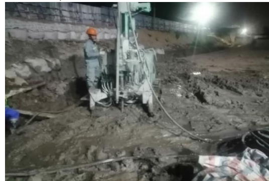
Fig.10. Start construction of the massive bottom plug hydraulic barriers
