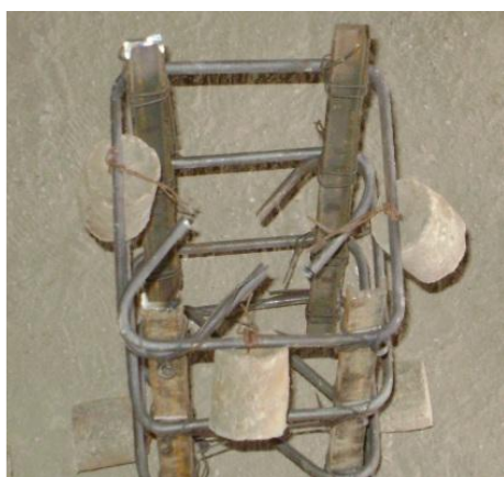
Fig 3. Channel reinforcement for casting
