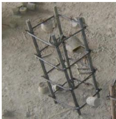
Fig 1. Normal reinforcement for casting
