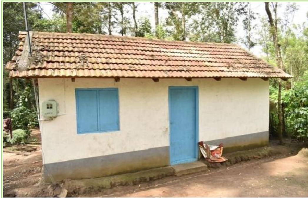
Fig 1.7:- Government provided Constructed house for Tribals.
