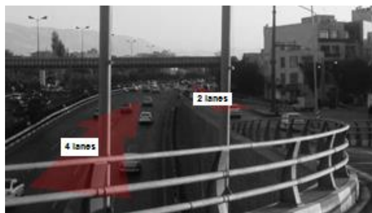
Figure 5. A view from the entrance ramp to Hemmat Highway (reduced lanes from 6 to 4)
