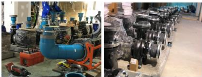
Figure 44: MareNostrum 5 heat exchanger, chiller and pumps
