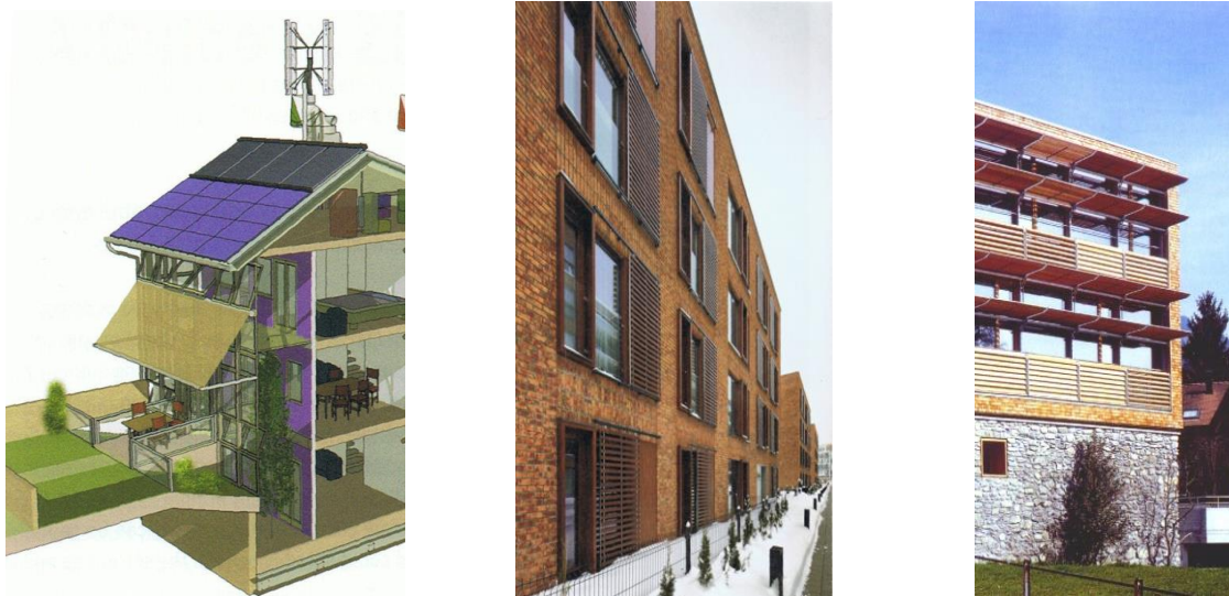
Fig. 43. Examples of various external shading systems to be applied over glazing in buildings; source [19].
