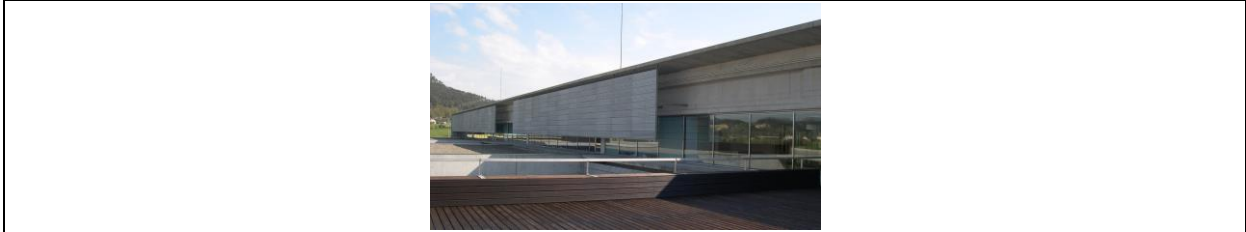
Figure 1: Metallic Shading device over a glazed façade in Labein-Tecnalia headquarters.
