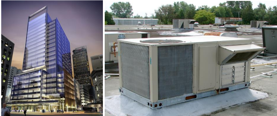
Figure 1: Glazed Multi-rise building (left) and rooftop HVAC systems (right)
