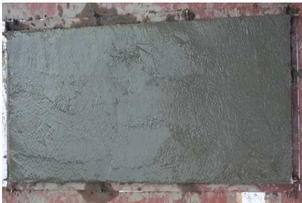
Fig.5 Ferrocement panel after finishing
