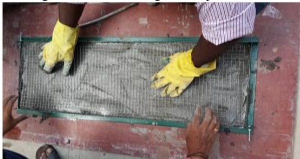
Fig.4 placing of wire mesh during casting
