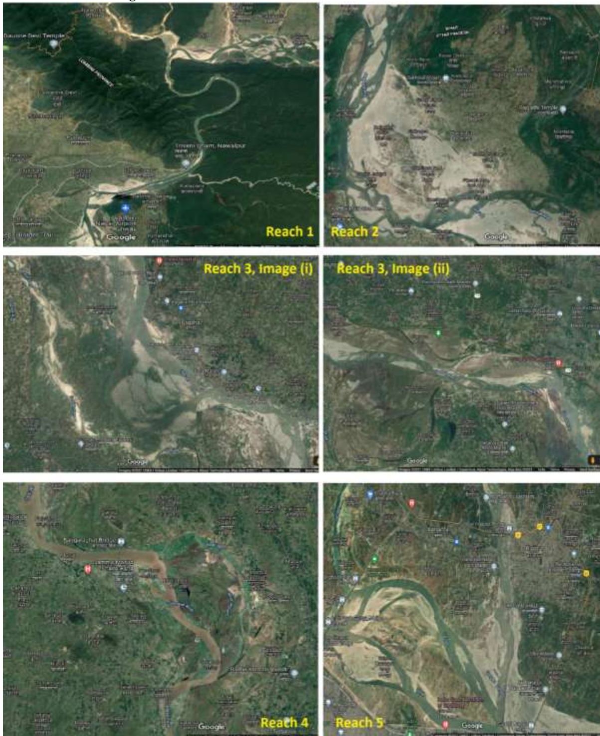
Figure 5:- Some Selected Views of Reaches of Lower Gandak River.
