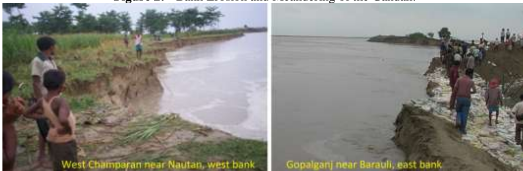
Figure 2:- Bank Erosion and Meandering of the Gandak.
