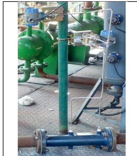
Figure 5. Venturi Flow Meter
