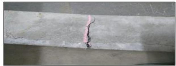
Fig. 2. Specimen after the failure in flexure test
