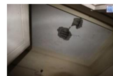
Figure 51 – (PD 03) GL 7: Toilet – Ceiling view
