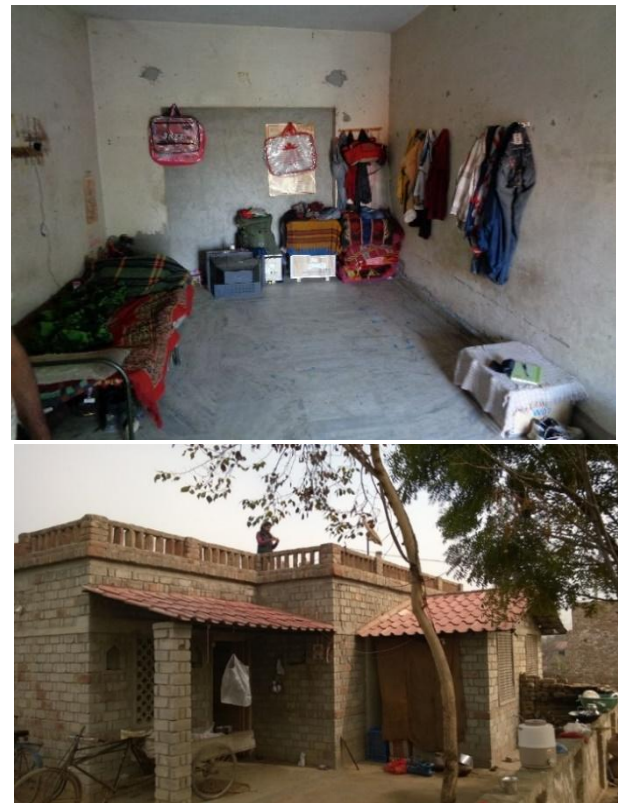
Fig. 3: EWS rented dwelling unit with on electric appliances for thermal comfort (left) and a recently constructed EWS house with perforated parapet wall. Source: author
