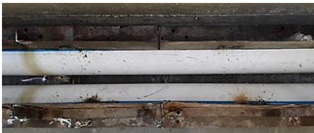
Fig. 5. Formwork of Slab Mold
