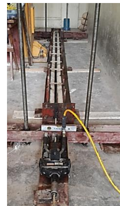
Fig. 8. Casting and Prestressing Setup
