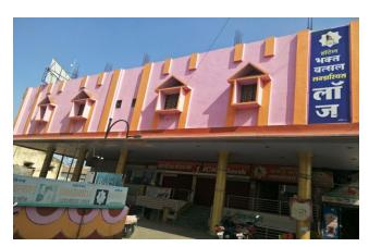
Fig.1 Front view windows with chajja and vertical fins (Site photograph)
