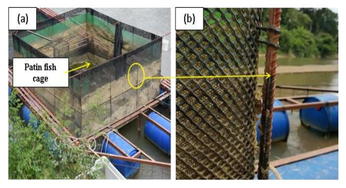
Fig. 4 (a) Patin fish cage made of y-bar steel in Temerloh, Pahang River, and (b) enlargement of y-bar steel structure of Patin fish cage.
