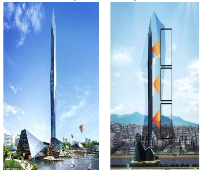
Fig 7: Infinity Tower (under construction in South Korea)
