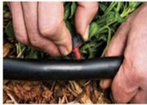
Fig. 19 Installation of drip nozzle into PVC pipe
