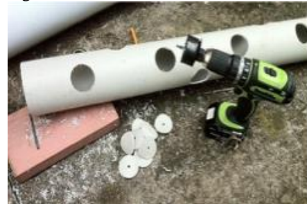
Fig. 20 Drilling of holes in the PVC pipe
