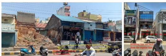
Fig. 10 Building Line not Maintained
