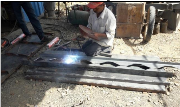
Fig. 5. Welding of Castellated Beam for hexagonal opening.
