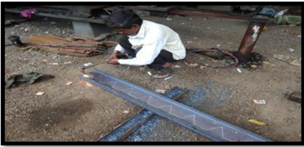
Fig.3. Marking and cutting the parent beam.
