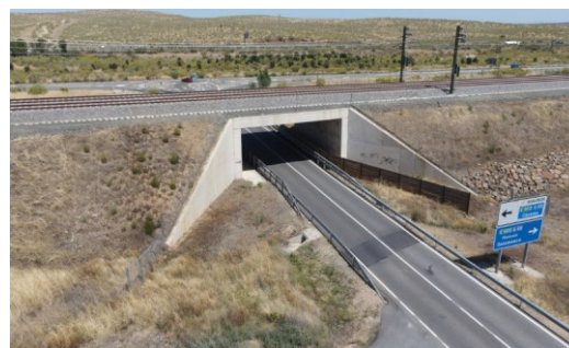
Figure 8: Underpass located at the 3 + 93 PK.
