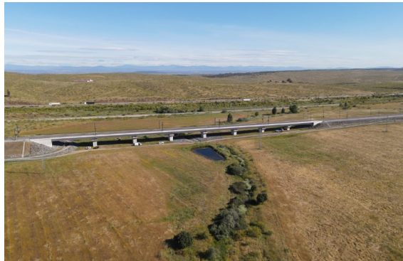
Figure 6: A viaduct formed of 8 simply supported beams. Its name is “Valdelinares”.
