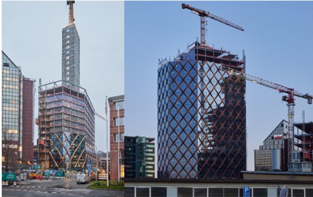
Figure 17: Kineum building demonstration project.
