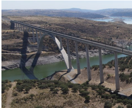
Figure 9: El Tajo Viaduct
