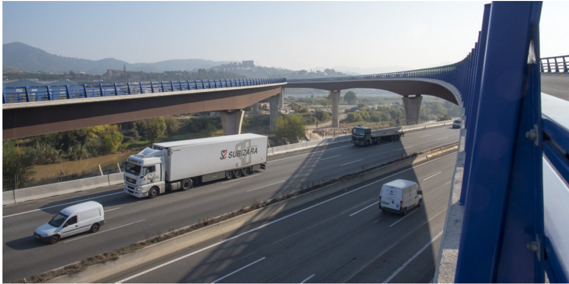
Figure 25: Bridge after construction.
