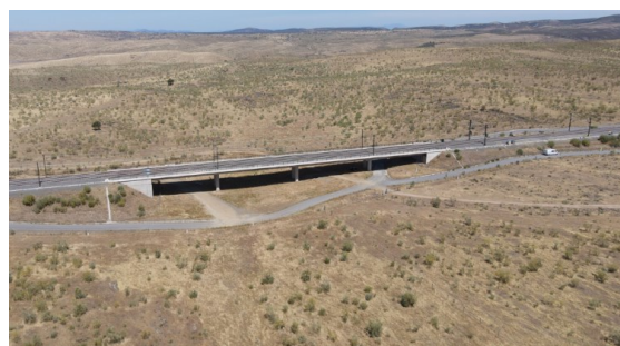
Figure 7: Viaduct formed of a continuous beam. Its name is “Viaducto de la Plata”.
