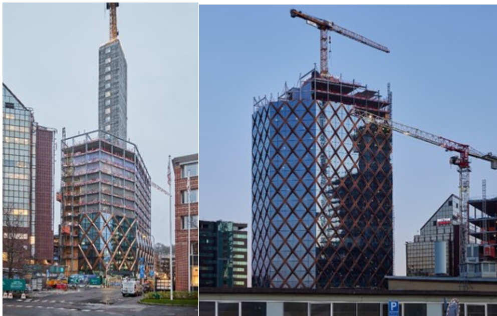
Figure 9 Construction process of Kineum project in Sweden.
