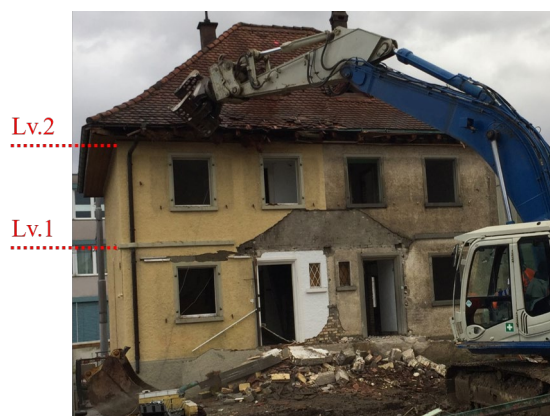
Figure 1. Studied building at the beginning of demolition.
