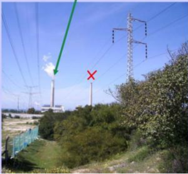
IEC Power Plant Ashkelon, Israel One FGD chimney (out of 8 in Israel)
