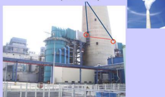
IEC Ashkelon Power Plant The connections to the chimney (FGD 2 units)
