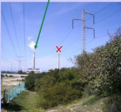
IEC Power Plant Ashkelon, Israel One FGD chimney (out of 8 in Israel)
