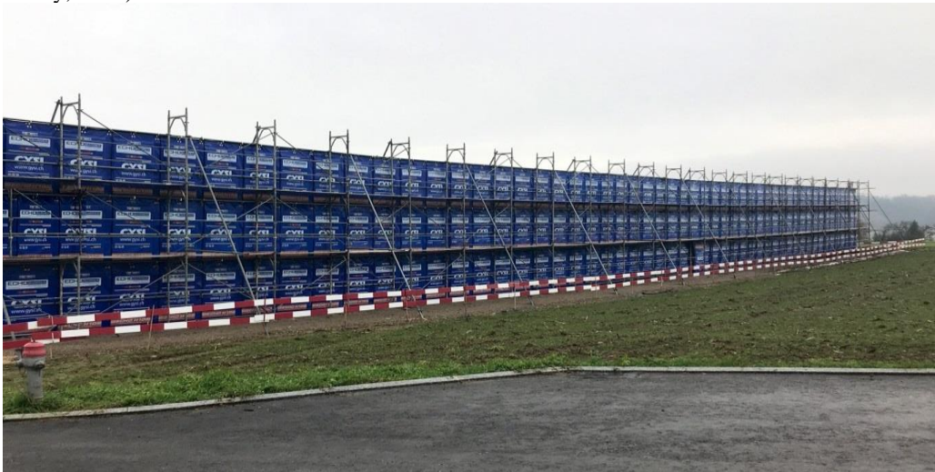
Figure 3: Mining Noise Control Management- Acoustic Barrier (blog.echobarrier.com)
