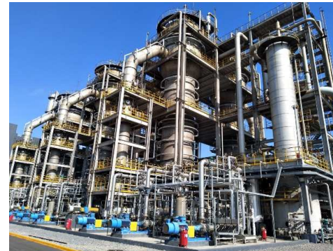
Lanzatech/Shougang Gas (CO/H 2 /CO 2 ) Fermenter Ethanol
