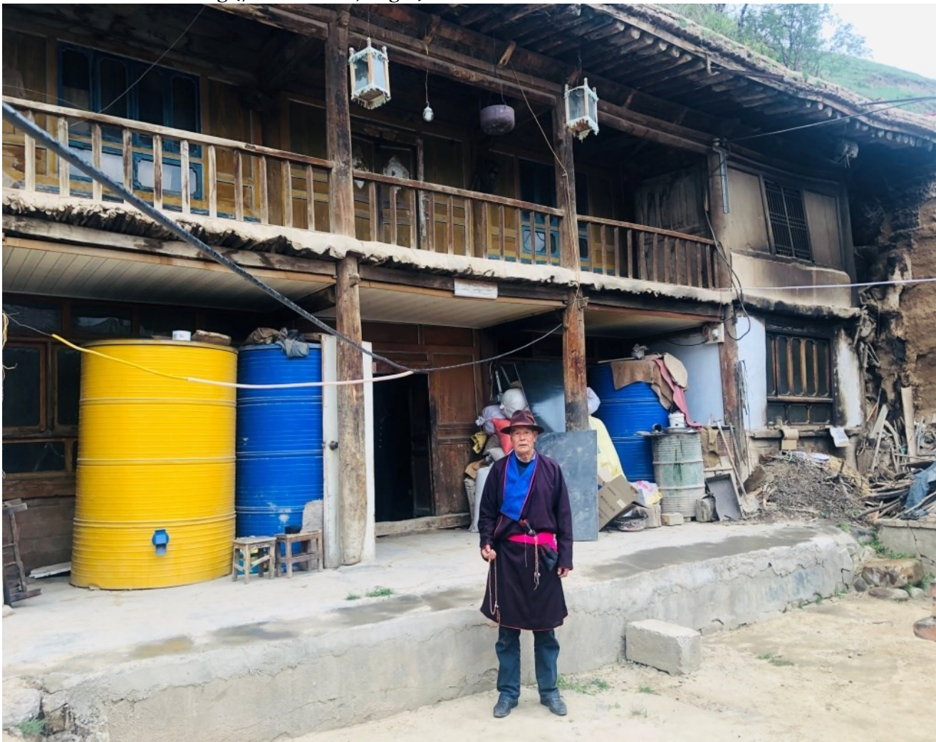
FIG 3. Wushisan in his home compound courtyard. The house is a 150-year-old traditional two-floored wooden building (7 June 2020, Jugui).
