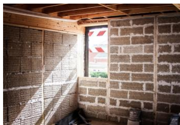
Figure 3. Hemp blocks for interior and exterior wall.
