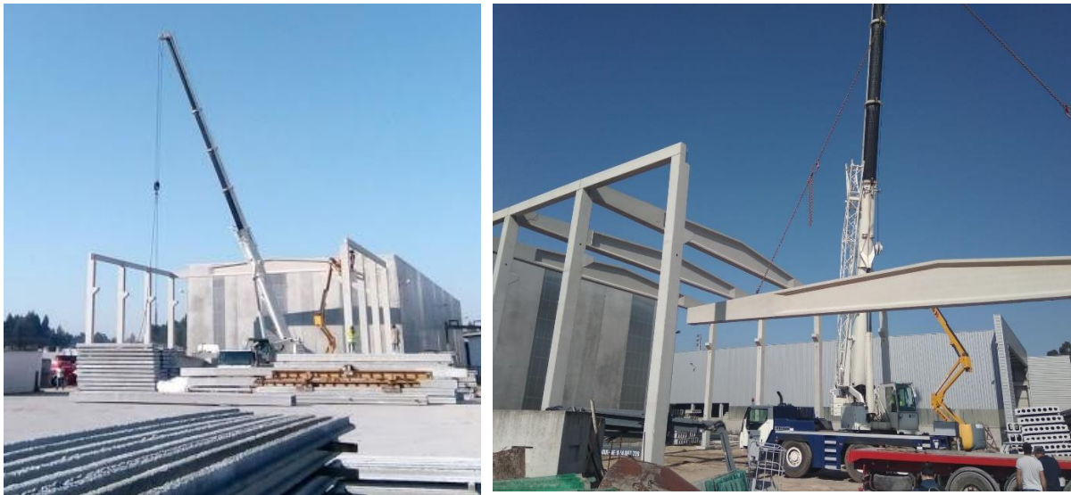
FIGURE 23. BEAMS PLACEMENT.
