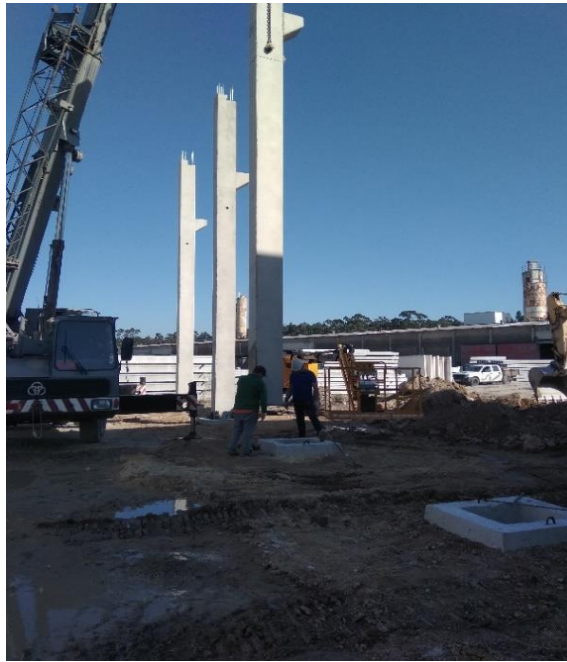
FIGURE 22. COLUMNS PLACEMENT.
