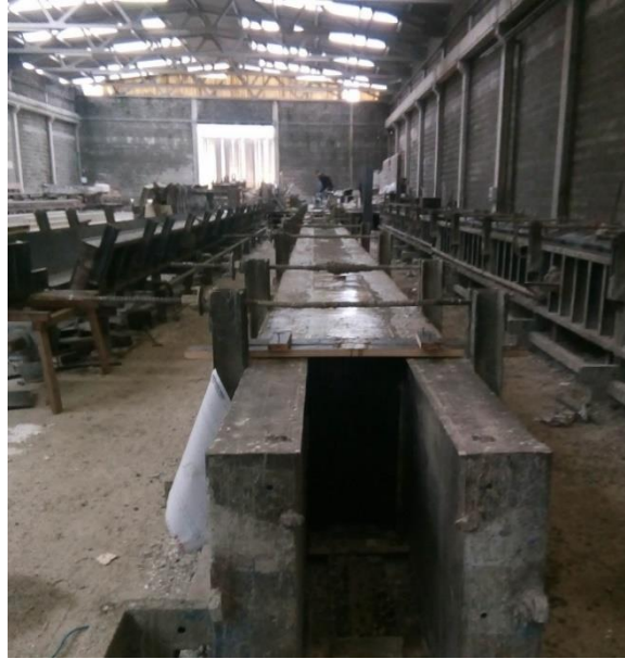
FIGURE 15. FRESH CONCRETE COLUMN DRYING AND HARDENING IN FORM.
