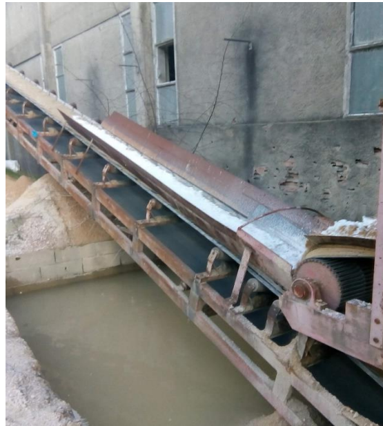
FIGURE 11. LIME ASH TRANSPORTATION TO CONCRETE MIXTURE.
