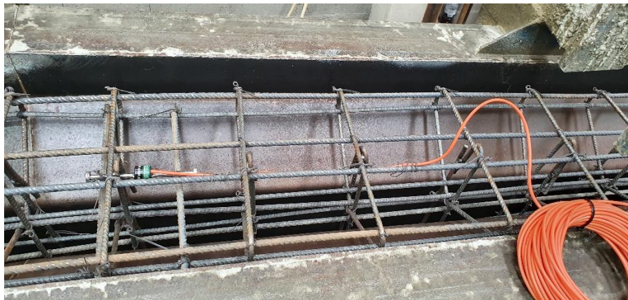
FIGURE 18. BEAM INTERNAL THERMAL SENSOR.
