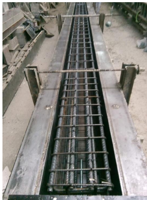
FIGURE 12. PRECAST CONCRETE COLUMN FORM AND REINFORCEMENT
