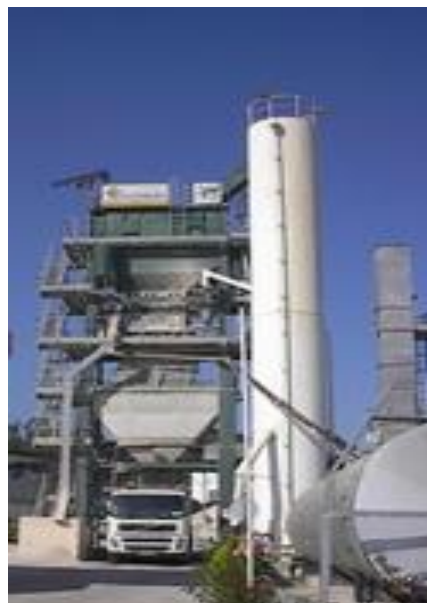
FIGURE 33. DISCHARGED BITUMINOUS MIXTURE TO A TIPPER TRUCK.
