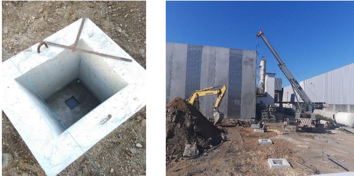
FIGURE 21. BASE FOR COLUMN.
