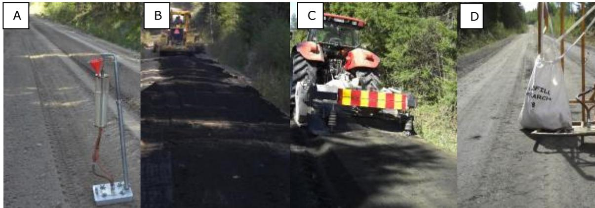
FIGURE 21. Examples of techniques of distribution, mixing and compaction from a road application, stabilizing of gravel road, Iggesund, where a) sieved till was distributed, followed by b) distributing green liquor dregs<sup>4</sup>, followed by c) mixing with a rotary mixer (milling depth 0,1 m) and finally d) the road after compaction.
