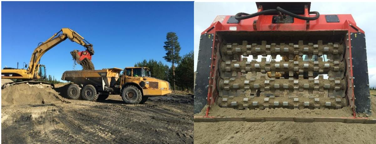
FIGURE 19. ALLU shovel. Round 2 of mixing by DH 4-17-X75. In the forefront, a batch of Ti/GLD after one round of mixing with bucket mixer is shown. Photo: Näsliden, Josef Mácsik.
