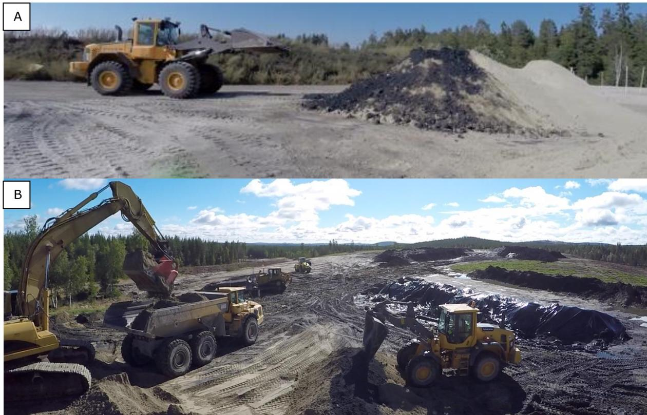
FIGURE 17. Pre-mixing by shovel. Pre-mixing is required before front shovel- and bucket mixing is performed. A) Pre-mixing Boden 2014, and B) pre-mixing and shovel mixing in Näsliden 2016.
