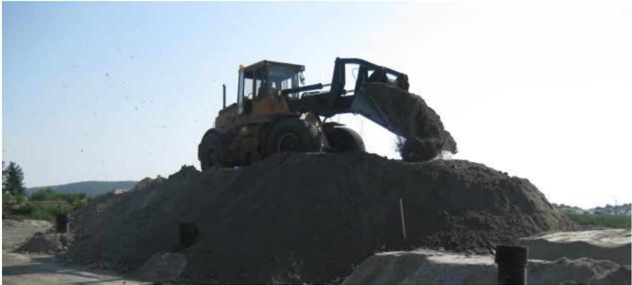
FIGURE 23. Distribution of protective layer formed by 0 - 150 mm till (Boden year 2014).
