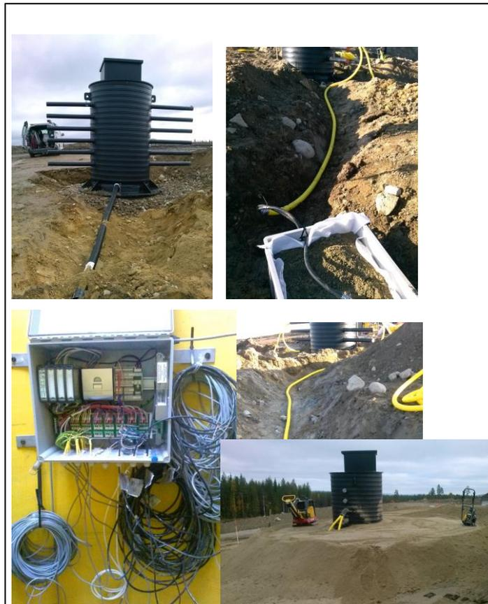
FIGURE 25. Sealing layer monitoring. Lysimeters installation.
