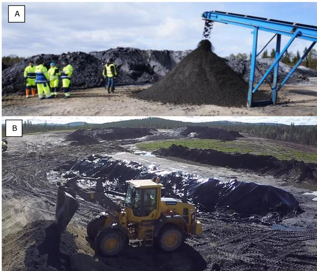
FIGURE 15. A) More than 2000 tons of GLD was stored from May 2013 to April 2014 (seen in the background). In the forefront Ti/GLD is being produced by forced mixer. B) Storage of GLD, covered by tarpaulin, during July-August of 2016, Näsliden. In the foreground, pre-mixing of Ti/GLD material is performed.
