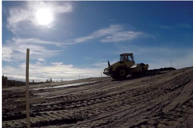
FIGURE 6. Compaction of the levelling layer (Näsliden year 2016).
