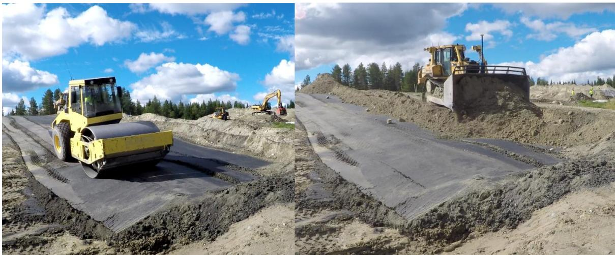
FIGURE 22. Compaction of the sealing layer in one step (final thickness 0.5 m) and distribution of protective layer by bulldozer. Distribution of the sealing layer material was performed similarly by bulldozer (Näsliden year 2016).
