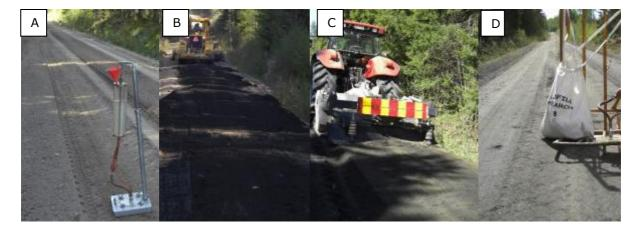
FIGURE 21. Examples of techniques of distribution, mixing and compaction from a road application, stabilizing of gravel road, Iggesund, where a) sieved till was distributed, followed by b) distributing green liquor dregs4, followed by c) mixing with a rotary mixer (milling depth 0,1 m) and finally d) the road after compaction.
