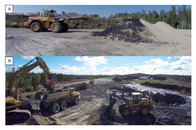
FIGURE 17. Pre-mixing by shovel. Pre-mixing is required before front shovel- and bucket mixing is performed. A) Pre-mixing Boden 2014, and B) pre-mixing and shovel mixing in Näsliden 2016.
