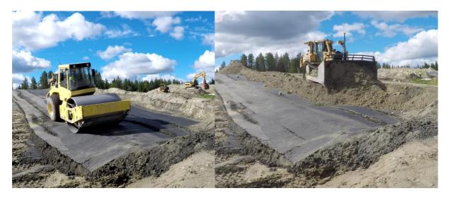
FIGURE 22. Compaction of the sealing layer in one step (final thickness 0.5 m) and distribution of protective layer by bulldozer. Distribution of the sealing layer material was performed similarly by bulldozer (Näsliden year 2016).
