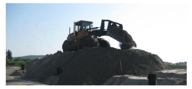
FIGURE 23. Distribution of protective layer formed by 0 - 150 mm till (Boden year 2014).
