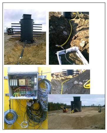
FIGURE 25. Sealing layer monitoring. Lysimeters installation.
