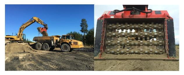
FIGURE 19. ALLU shovel. Round 2 of mixing by DH 4-17-X75. In the forefront, a batch of Ti/GLD after one round of mixing with bucket mixer is shown. Photo: Näsliden, Josef Mácsik.
