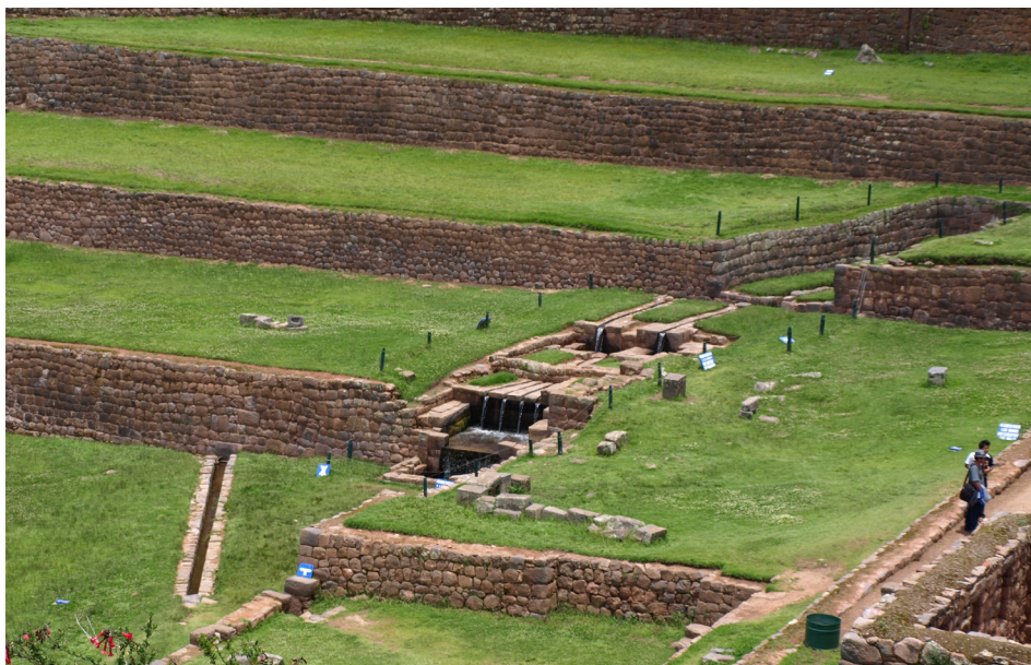
Figure 7. The perfect trace of walls and channels of the Inca ritual site of Tipón (photo by Timmi Tillmann).
