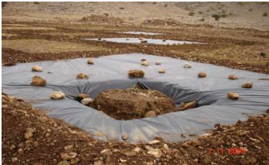
Fig. 9. Plastic Mulch Application to Collect Rainwater and Erosion Control
