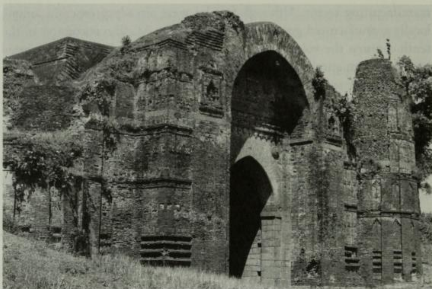
Fig. 14. Dakhil Darwaza (ca. 1433–59), seen from within the citadel of Gaur.
