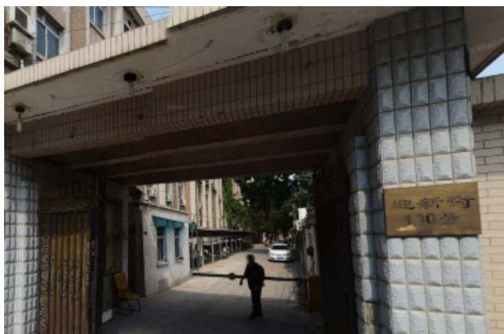
Main entrance of the Institute, 100 Yingxin Street—2020
