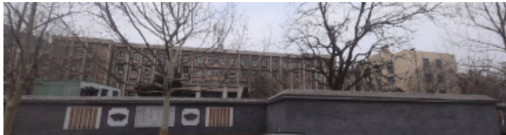
5-storey building of the Institute where the leak happened, source: Baidu
