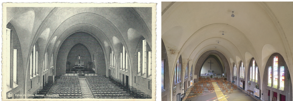
Figure 13. Church of Divin Sauveur; Left: Before the extension (Photo: Willy Balasse, in https://www.delcampe.net ); right: After the extension (Photo: Authors, 2020).
