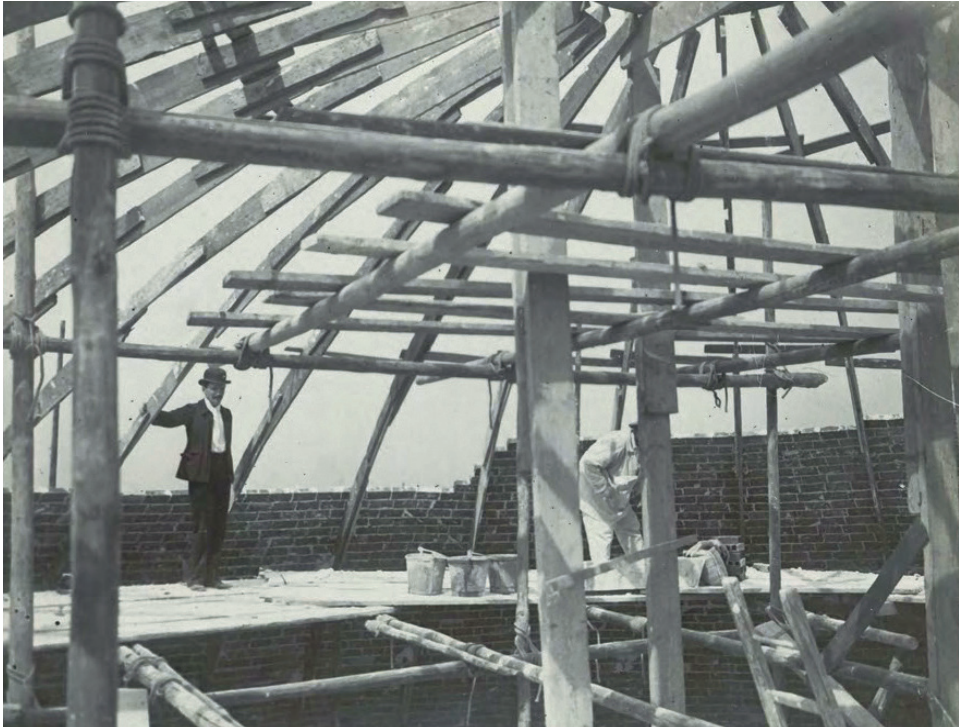
Figure 7. Dome of the Petit Palais under construction (Girault 1908).
