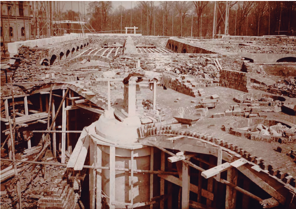
Figure 9. Vaults of the basement of the Petit Palais under construction (Girault 1908).
