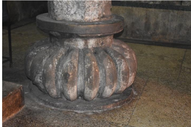
Figure 7 Amalaka Pillar base
