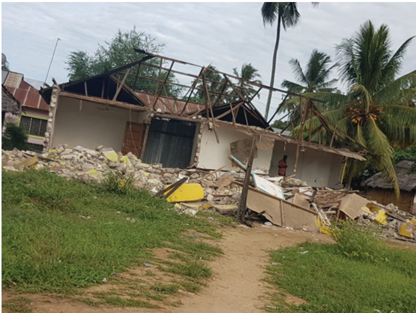
Figure 5.2 Remnants of a house partly built on governmental land
