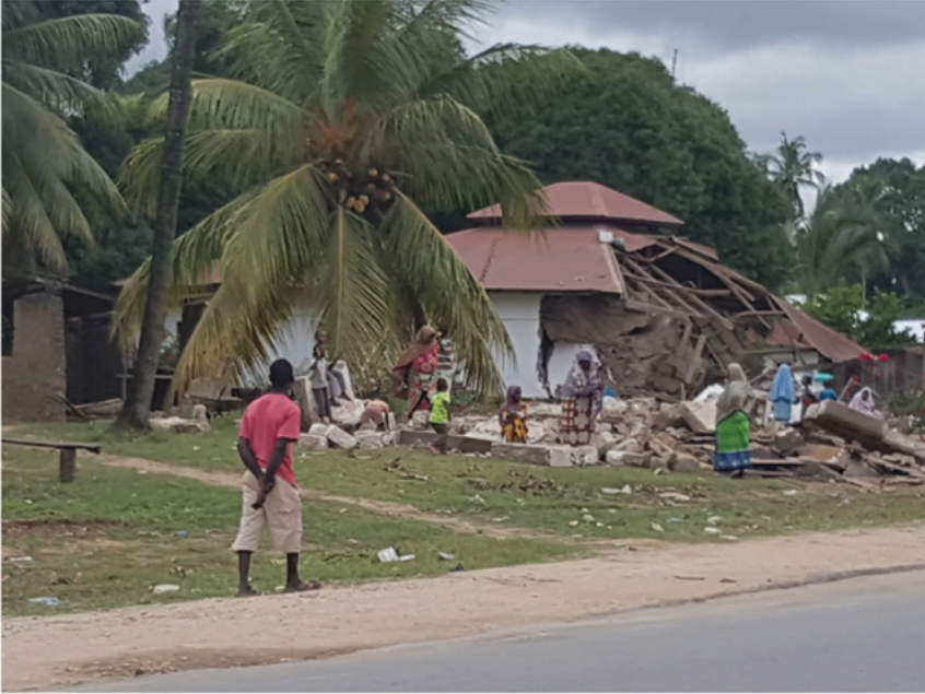
Figure 5.3 Remnants of another house partly built on governmental land
