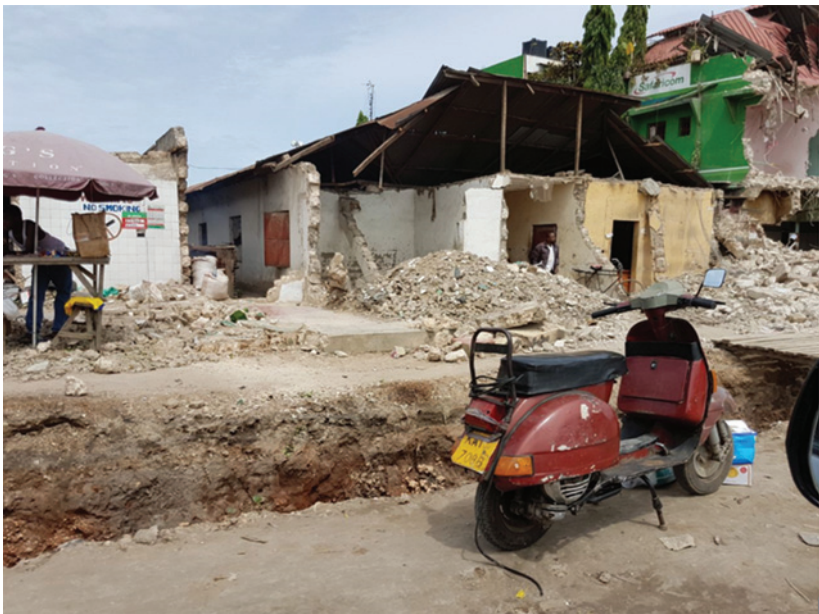
Figure 5.6 Demolition of homes
