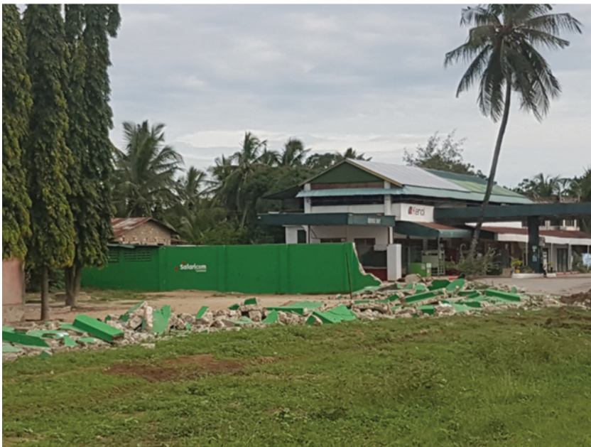
Figure 5.4 Demolished by bulldozers: the wall of a school in Tiwi
